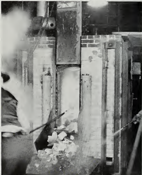
Pulling a charge of coke from the Survey's experimental oven.
